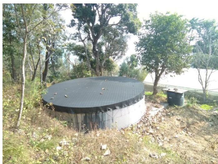
Figure 3.1: Water Storage Tanks
